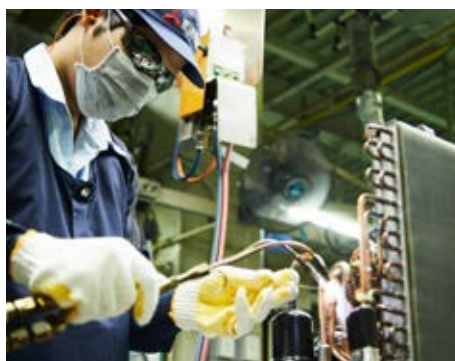
Pipe brazing by experienced professionals
